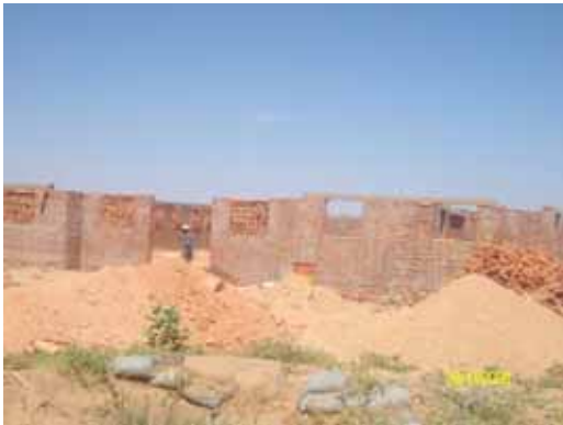
El Jeneina church under construction
