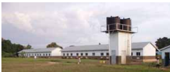
The classrooms and water tower
