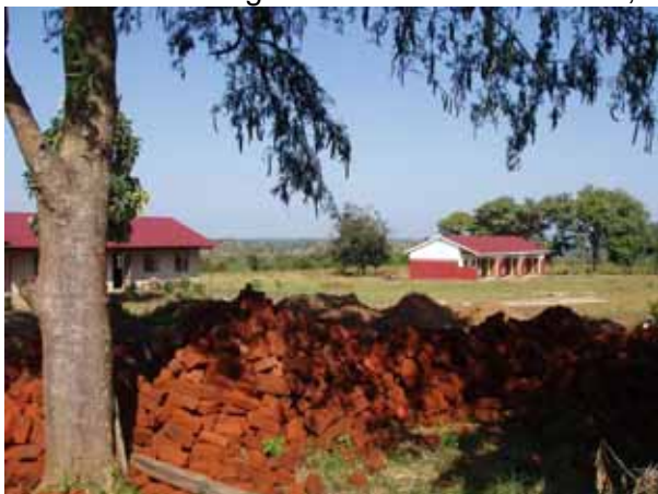
CBPC - a beautiful new college still under construction
